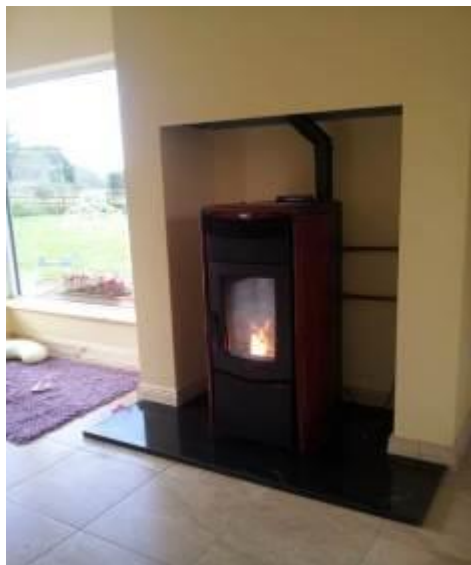
Figure 20: Typical stove/boiler inset into existing fire place
