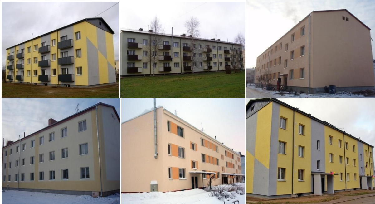
Figure 24: Buildings in Ozolaine village (Limbazi region) after the renovation
