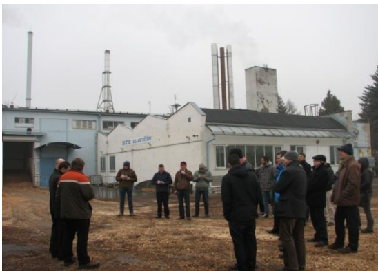
Figure 4 Welcoming at Malé Pole boiler house in Slavičín
