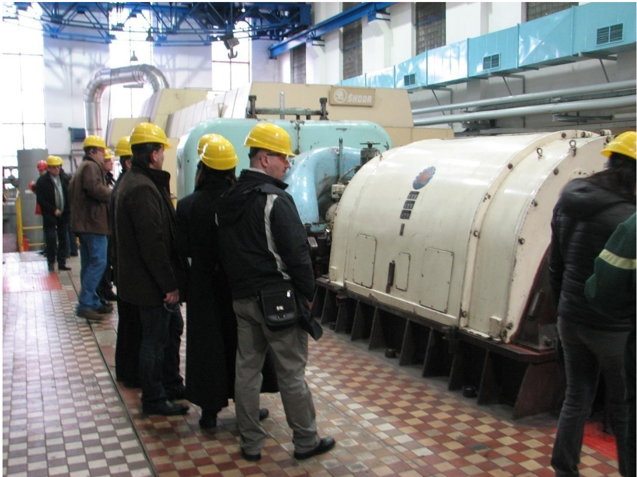
Figure 2 Study visit to the boiler house of DHS in Zlin
