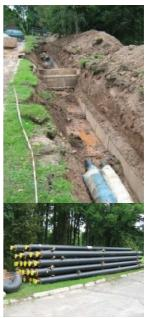
Fig.2.4. Reconstruction of heat distribution pipes in Limbazi in summer 2011
