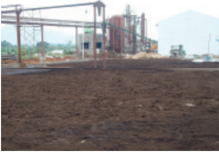
BIOMASS GASIFIER PLANT
