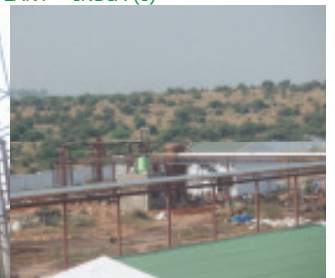
GENERAL VIEW BIOMASS GASIFICATION PLANT
