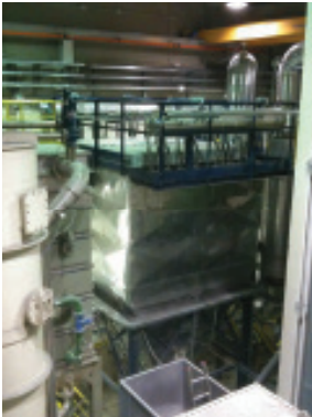
HIGH TEMPERATURE SYNGAS FILTER
